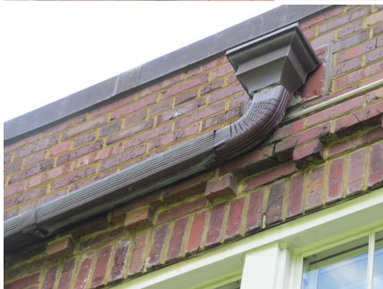
Copper scupper and downspout
