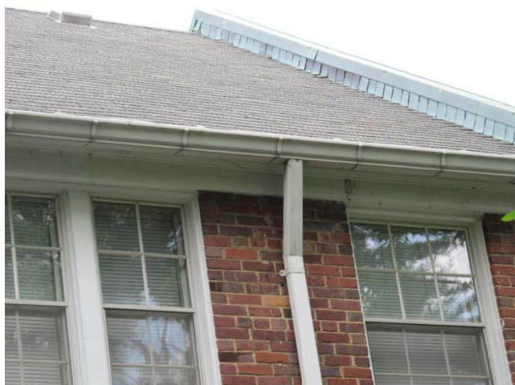
Metal gutter and downspout
