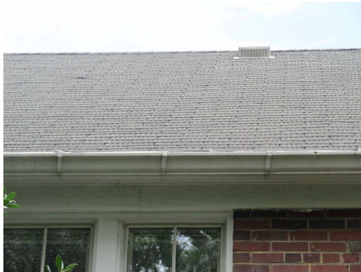
Asphalt shingle roof
